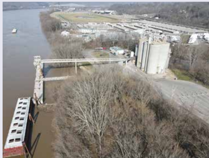
Anderson sold land to allow for the staging area at Cargill, which increased safety and reduced traffic backups on Kellogg Avenue.
