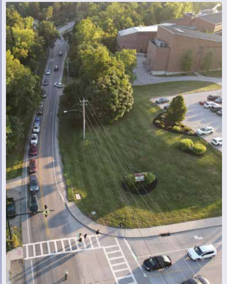
The Bartels Road sidewalk will be completed this year.
