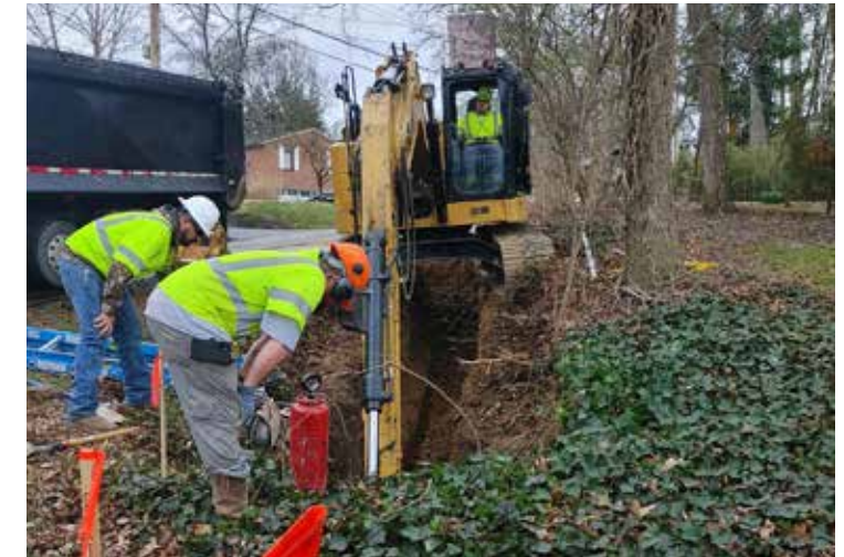
Construction on the Paddison Road sidewalk is underway.
