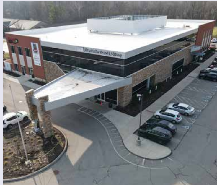
Professional Center of Anderson office building
